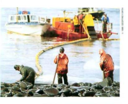
Above-A vessel-mounted belt skimmer collects oil dislodged from the rocky shore by workers wielding high pressure water sprayers. Containment boom keeps the dislodged oil from spreading seaward. Below-Workers use water spray to wash oil into the sound where it is sucked up by vacuum equipment.
